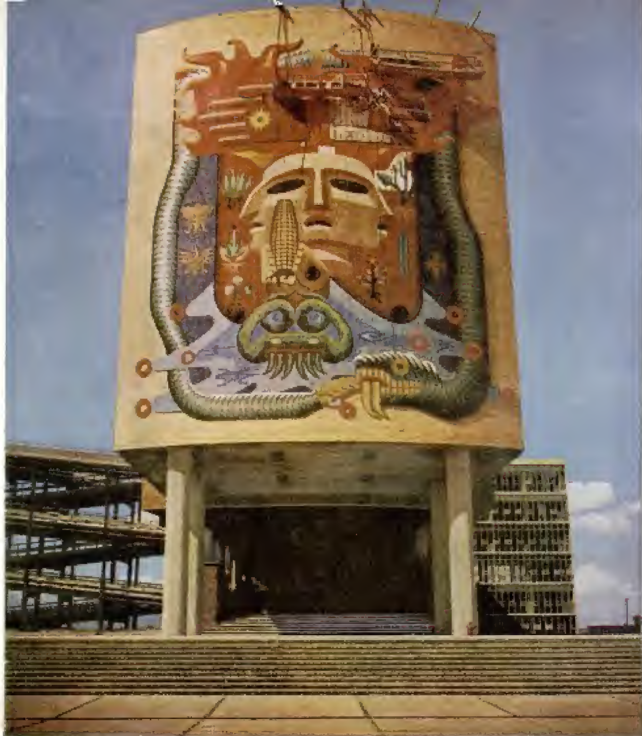
Artists worked from scaffolding on medical building. Aztec mosaic of glass tiles depicts Life and Death
